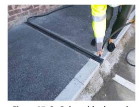
Figure 27: OxGul-e cable channel
